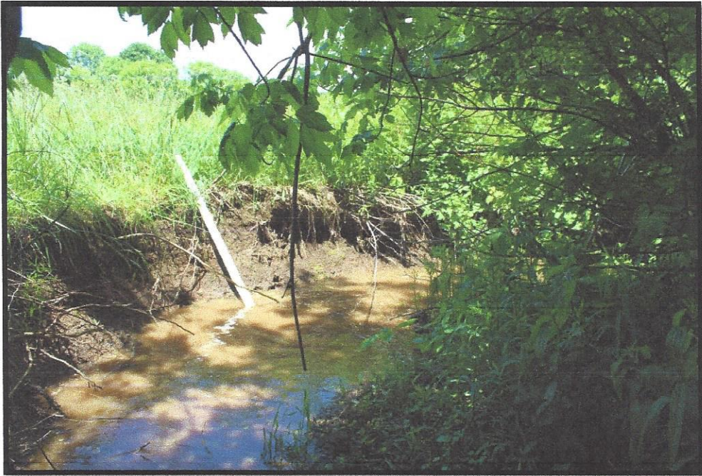
Photo 6 – Bank erosion and sedimentation
