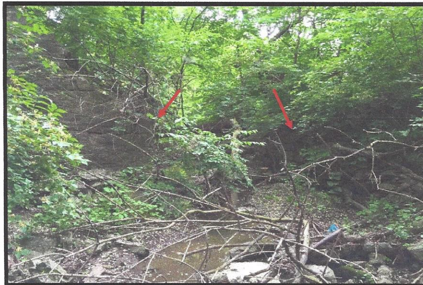
Photo 12 - Stone abutments along old railroad crossing at upstream end of Reach 2B
