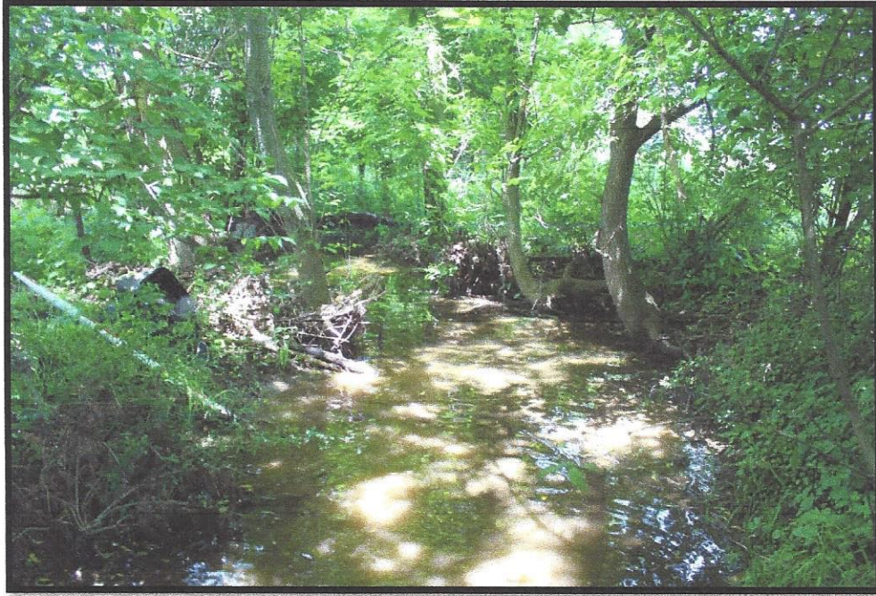
Photo 9 – Bank erosion and undercut trees
