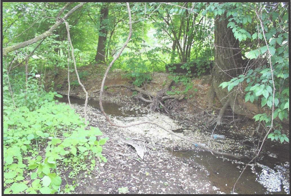
Photo 5 – Bank erosion, undercut tree, small debris jam and sedimentation
