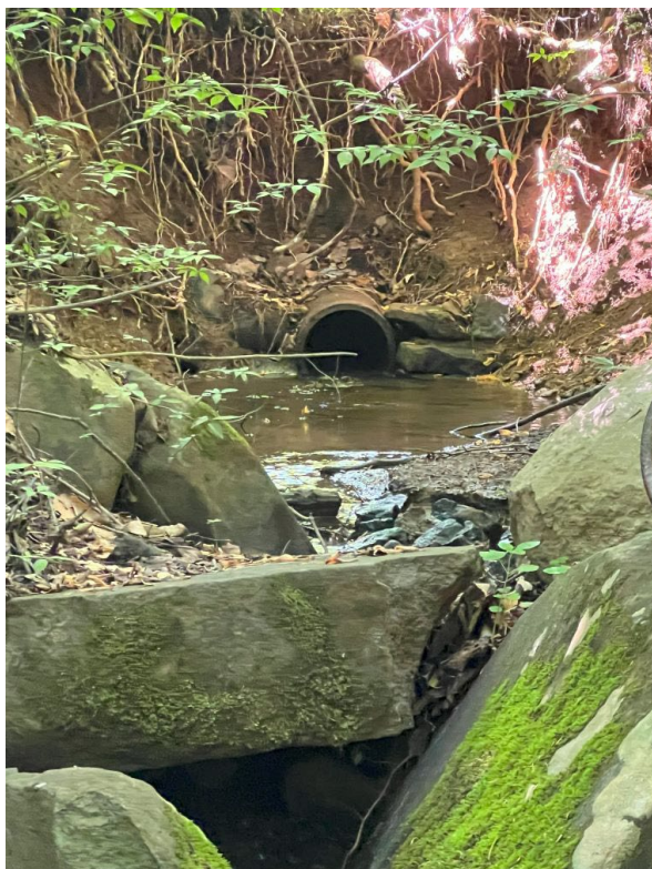
Photos 9 and 10 – Drain pipe at base of head-cut with boulder revetment in foreground
