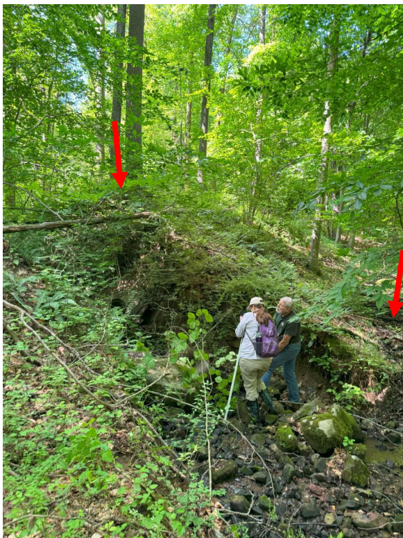
Photos 7 and 8 - Pond embankment (red arrows) with breach and severe head-cut (exposed drain pipe)
