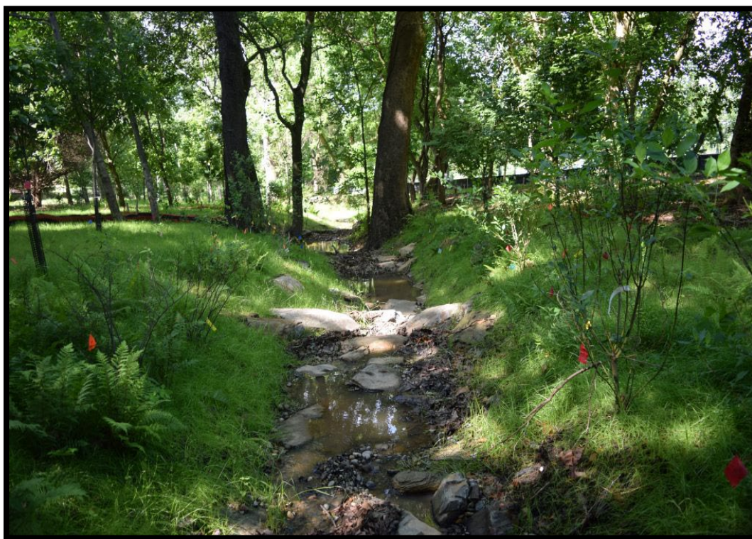
Photo 12 – Example of Constructed Timber Boulder Step Pools
