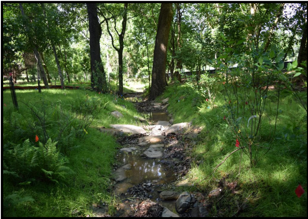
Photo 15 – Example of Constructed Timber Boulder Step Pools
