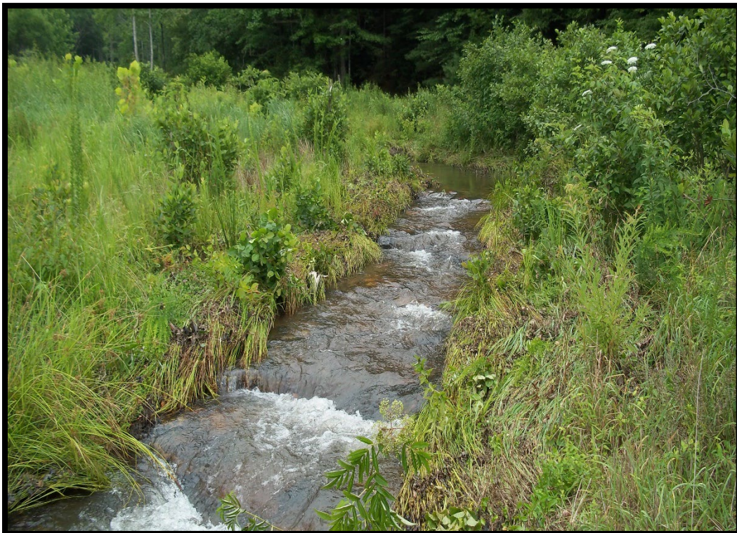
Photo 13 –Example of Constructed Boulder Cascade
