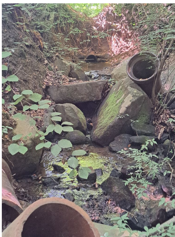
Photos 9 and 10 – Drain pipe at base of head-cut with boulder revetment in foreground
