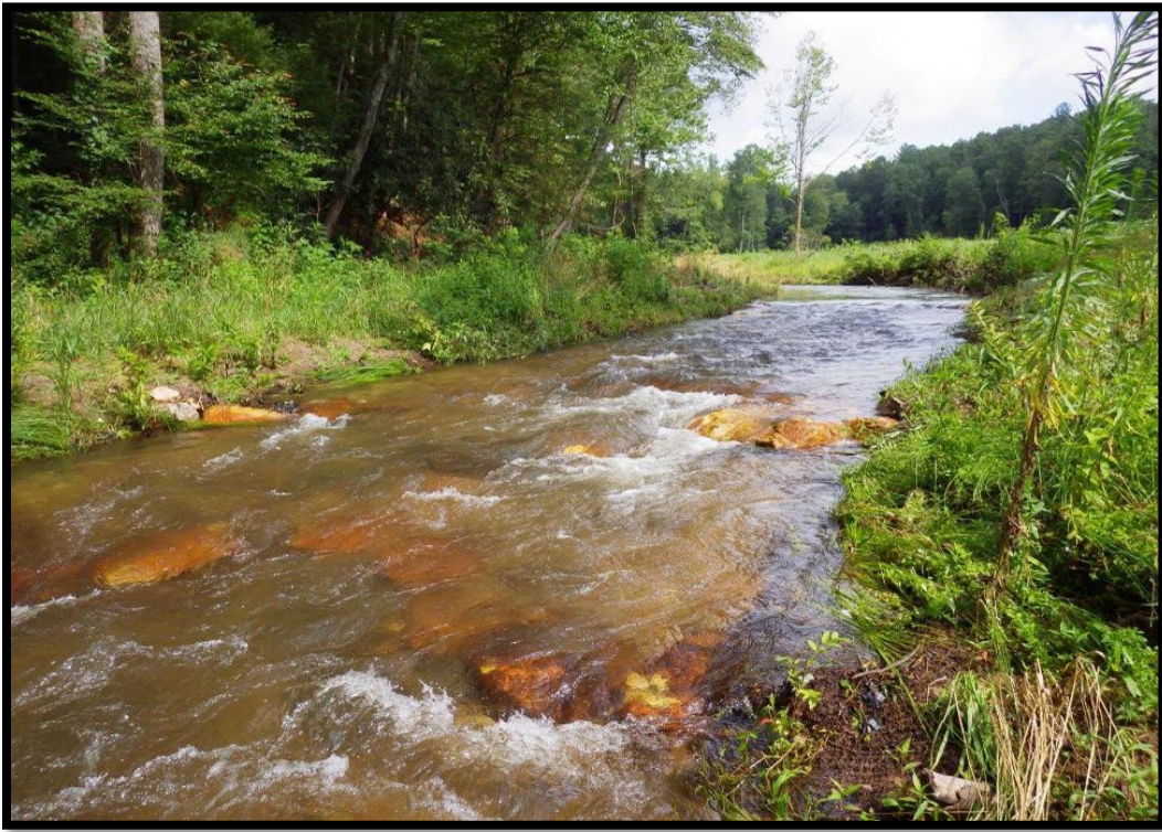
Photo 14 –Example of Constructed Boulder Cascade
