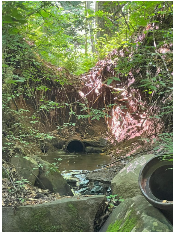
Photos 7 and 8 - Pond embankment (red arrows) with breach and severe head-cut (exposed drain pipe)
