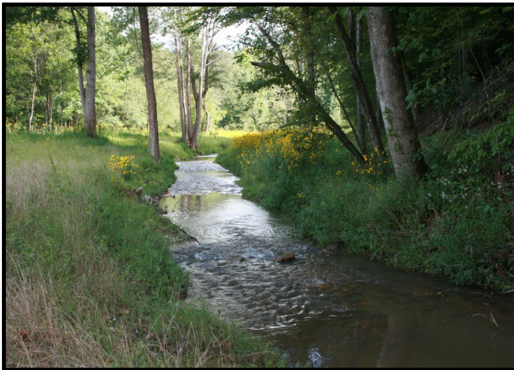
Photo 17 – Example of Constructed Riffle-Pool Sequence
