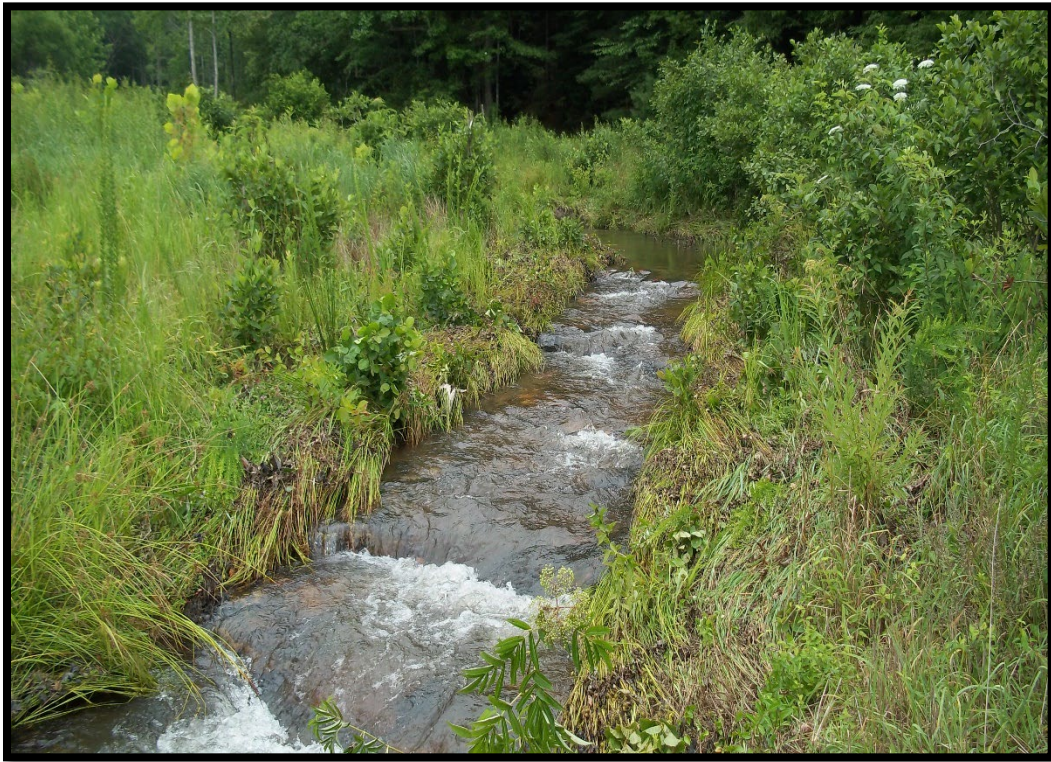
Photo 13 –Example of Constructed Boulder Cascade
