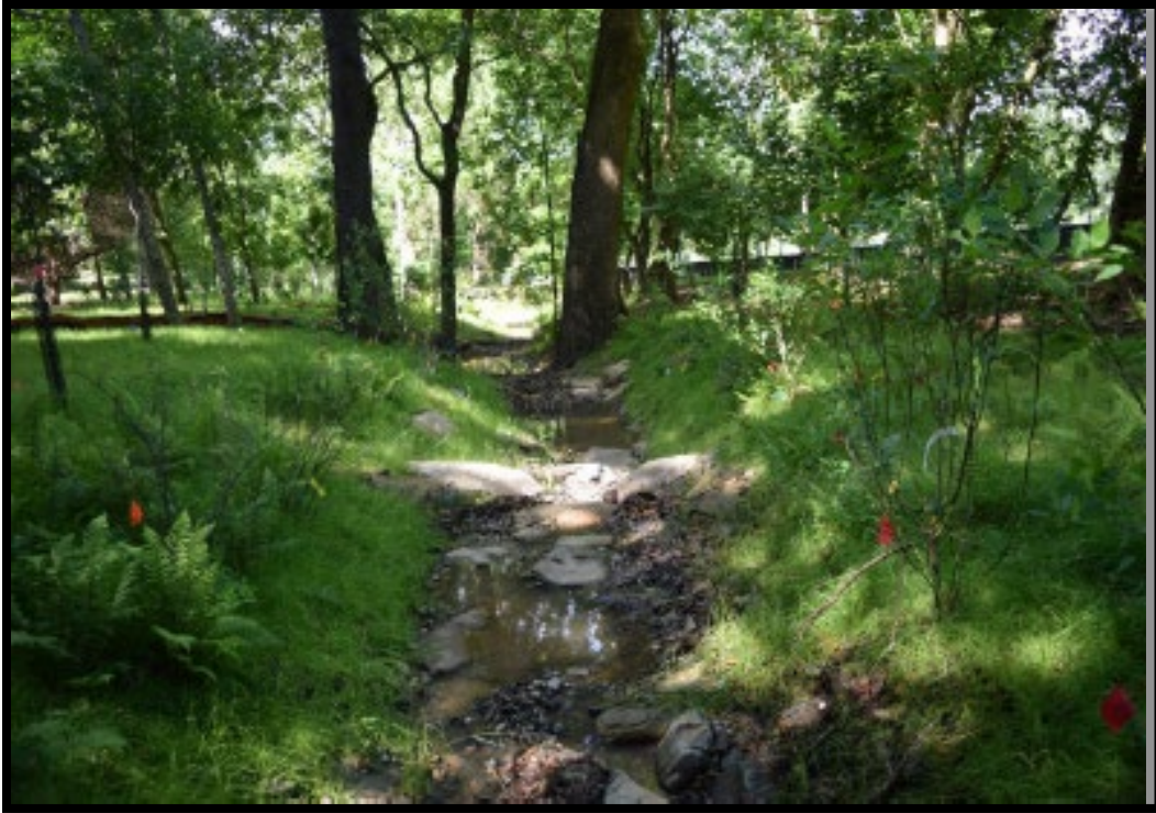
Photo 12 – Example of Constructed Timber Boulder Step Pools
