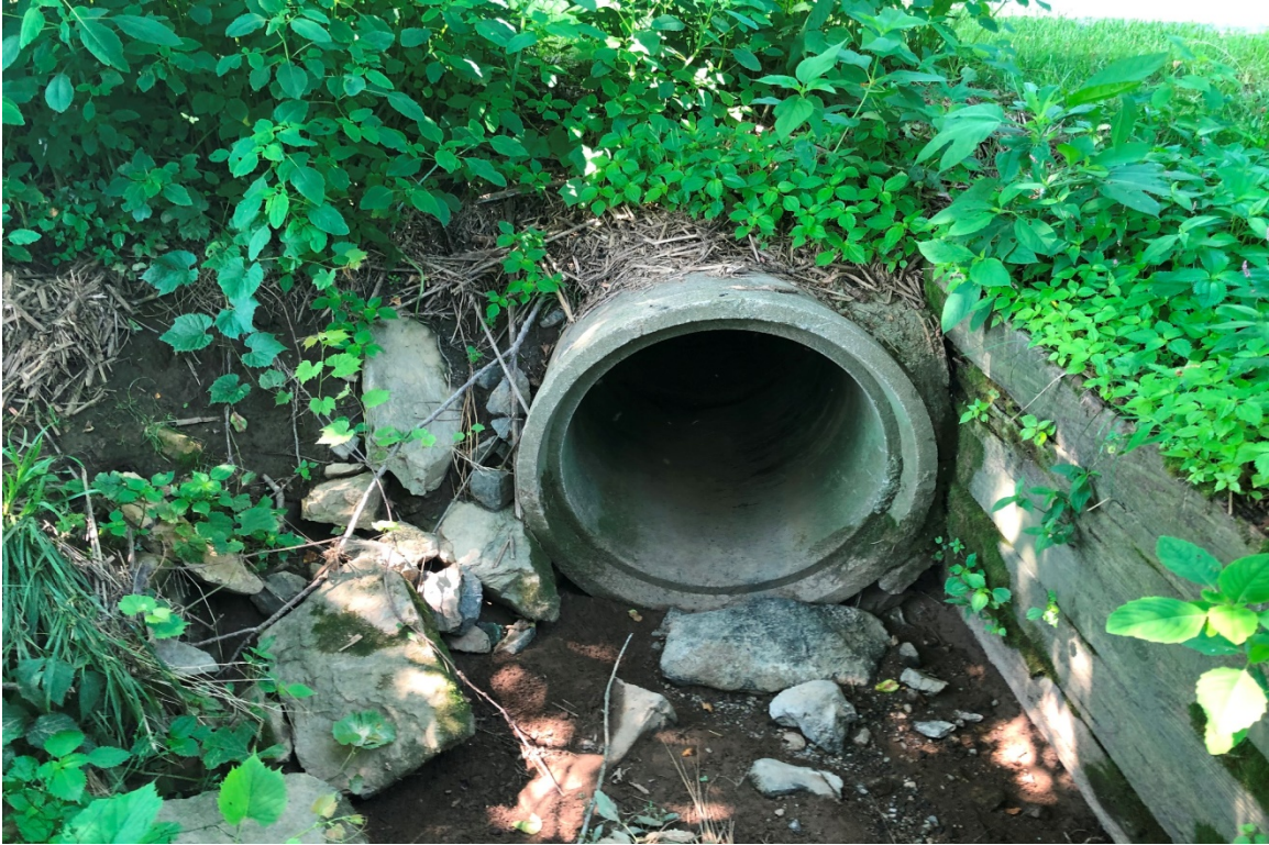
Inlet of culvert pipe under Culvert Road that carries runoff from fields
