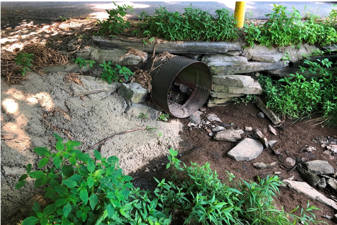
Outlet of culvert pipe under Culvert Road that carries runoff from fields
